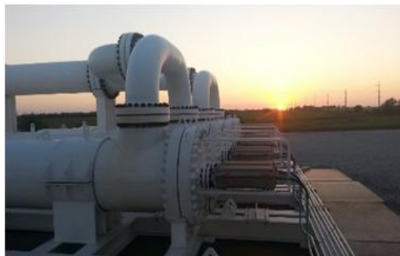
Fig. 1: Industrial design schematic and photo of AOT four-vessel viscosity reduction system. Following fabrication and pressure testing, this 110-ton unit was ASME-certified, approved for use in hazardous location Class 1, Div. 1. rated areas, and installed on a 500,000 barrel per day mid-continent pipeline operated by a $36 billion North American energy company.
